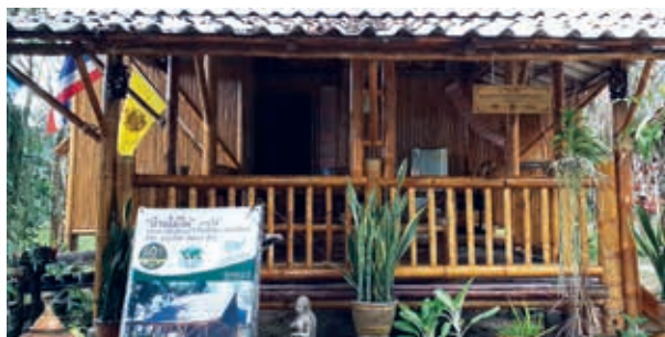
A bamboo house constructed during hands-on training in February 2012 in Phang Nga Province, Thailand, as part of a project that assessed the physical properties of five bamboo species for their suitability and use for furniture-making and house construction in tsunami-affected areas in Thailand. Photo: H. Ok Ma, ITTO
