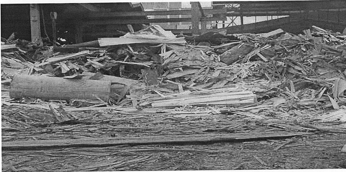
Photo: Residue ready for boiler.
