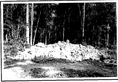
Photo No. 19 Blocking of road with filling materials
