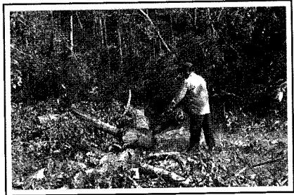
Photo No. 21 Cutting/Cleaning of logging debris
